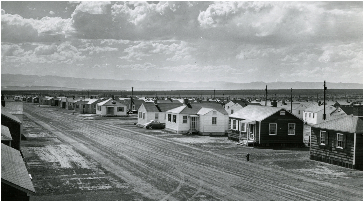
Houses built in Dragerton long after the 1922 strike
